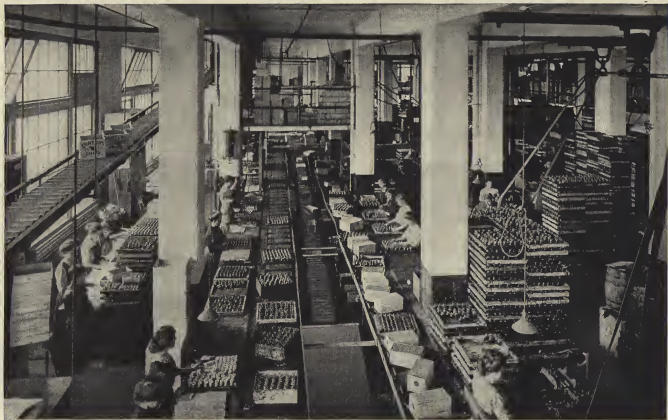
General View of one side of Bottling Floor.
